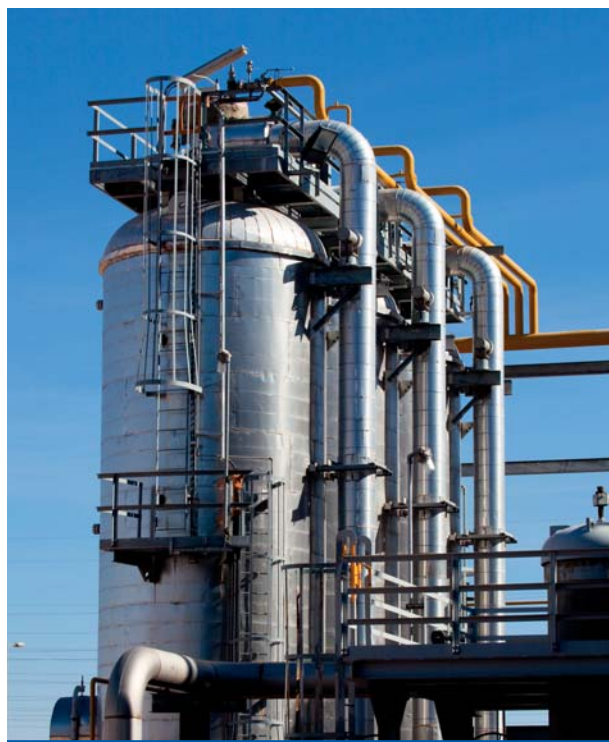
Gas reinjection project, Algeria
