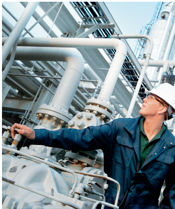
Engineer at Tioga Gas Plant, North Dakota
