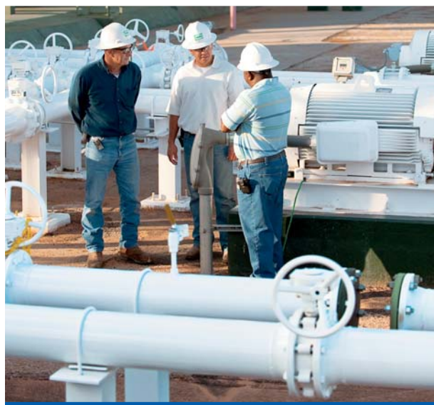
Seminole Gas Plant, Texas
