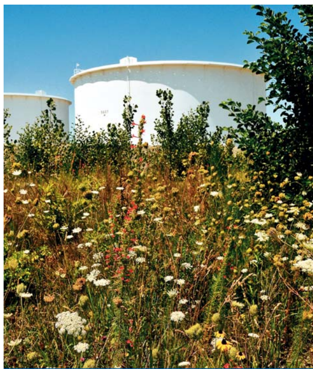
Remediation project, Chesapeake, Virginia
